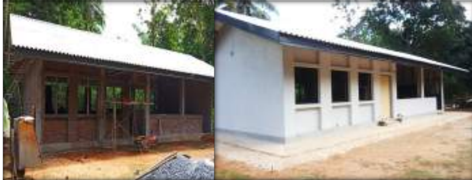
Construction of a building for the Imbulgolla Dambagahamuduna Primary School - Allocated amount Rs. 7,500,000.00
