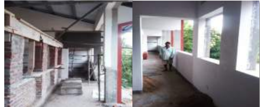
Renovation of the Nabadagahawatte Al-Rahuman Primary School Allocated amount – Rs.4,000,000.00
