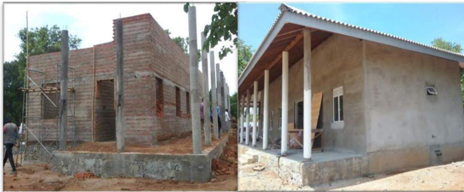
Completion of work at Laggala Depot Allocated amount -Rs. 20,000,000.00
